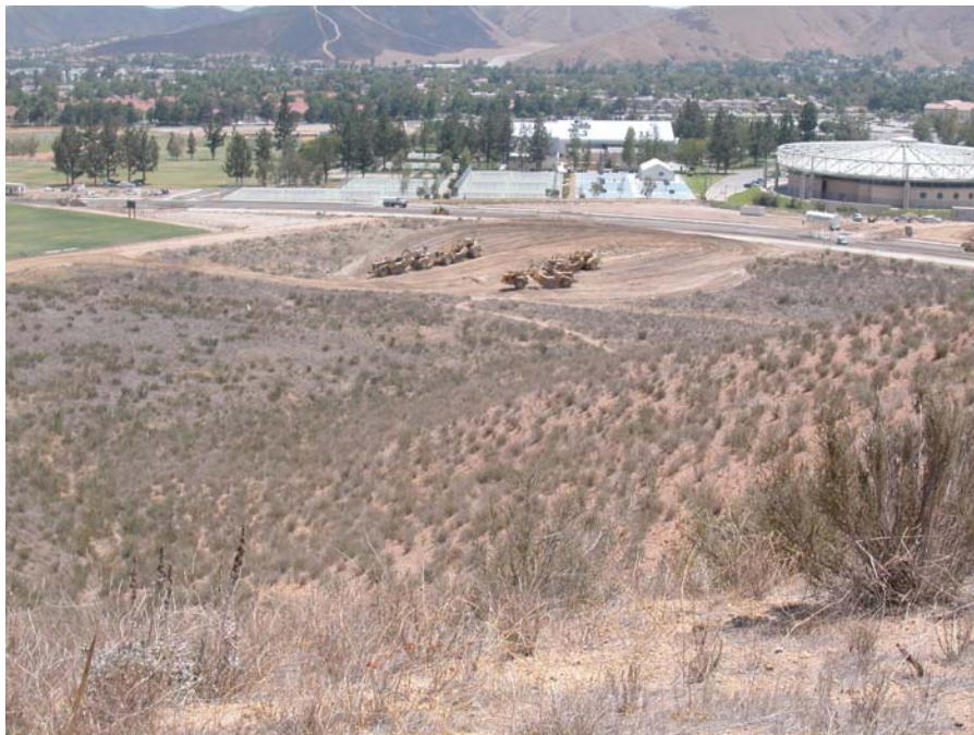
Figure 2. Removal of spoil, summer 2007.
