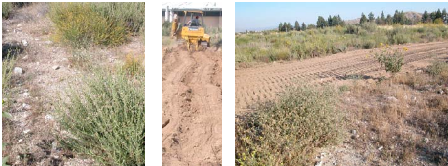
Figure 7. Breaking up compacted soil.
