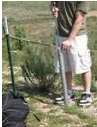
Figure 4. Sliding hammer placed over the rebar and raised, before first hit.
